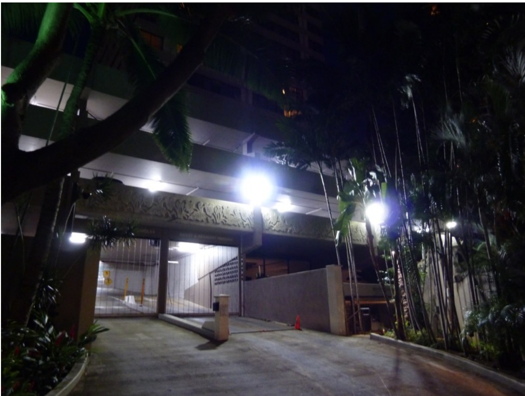
The Windsor condo in Hobron Lane is one of the worst examples of excessive and abusive LED over-illumination of its garage levels & front entrances - “like a prison yard”.
